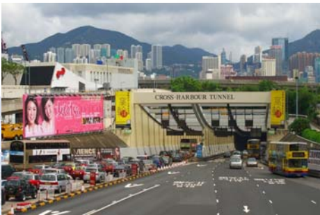
First BOT tunnel in HK, opened 1972, one of the most successful BOT projects (Source: Kowloon Motor Bus, 30X/230X, 2008)
