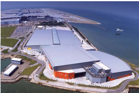
First proper PPP project in HK, opened 2005 (Source: Asia World Expo, 2008)
