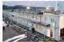
Temporary hospital in Wuhan constructed using MC technology
