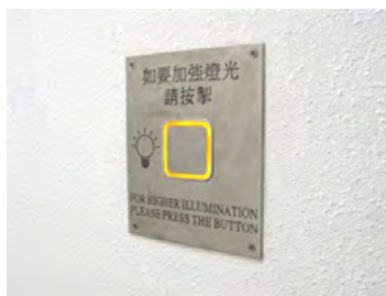
Manual push button of two-level lighting control
