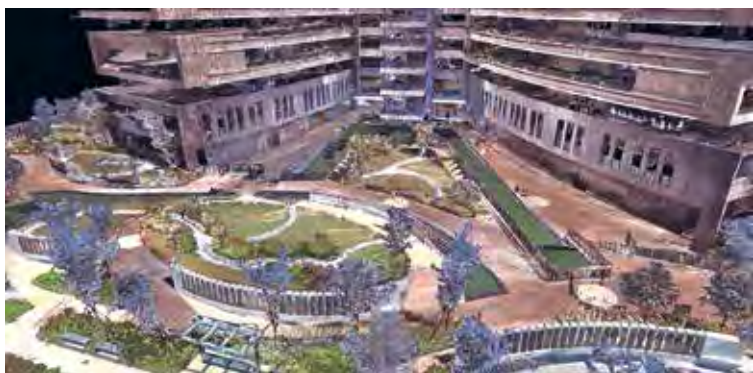
UAVs enable project management and site progress monitoring through precise geospatial models/pointcloud.
