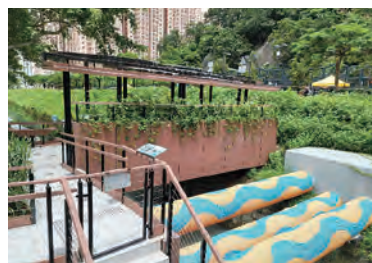
Viewing Platform above the Nullah
